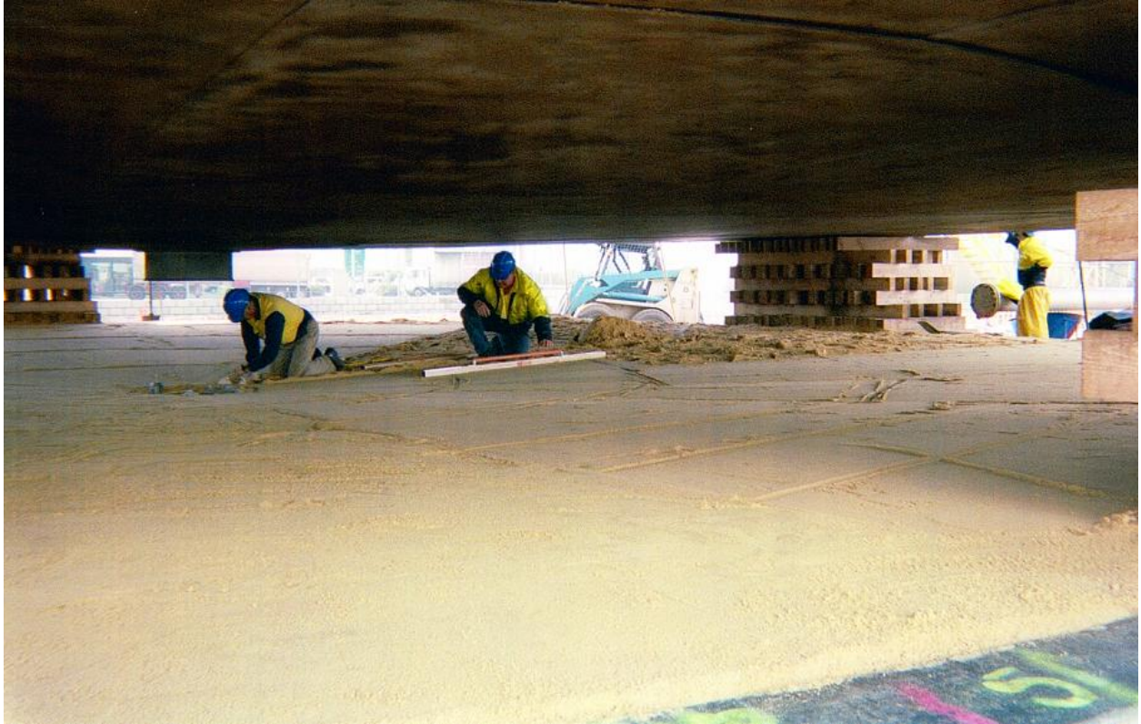
FIG 5 Profiling Foundation BP Kewdale
