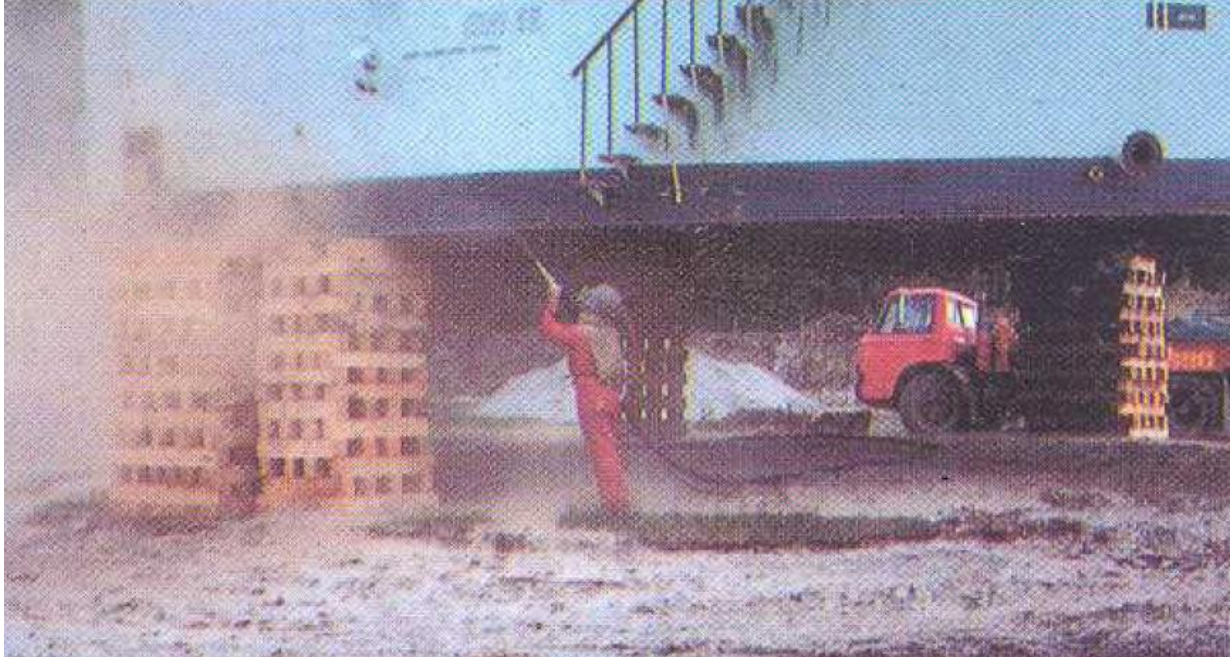
FIG 3 – Grit Blast prior to inspection and coating of underfloor
