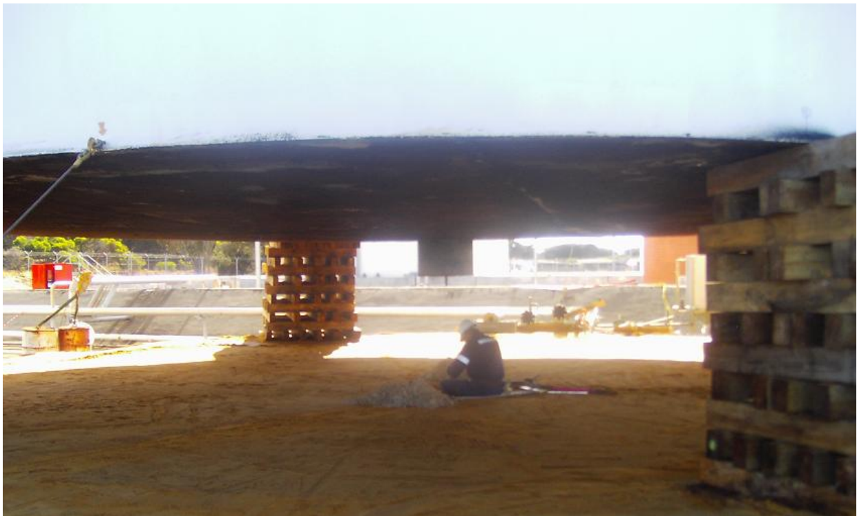
FIG 6 Installation of Leak Detection Sump HMAS STIRLING
